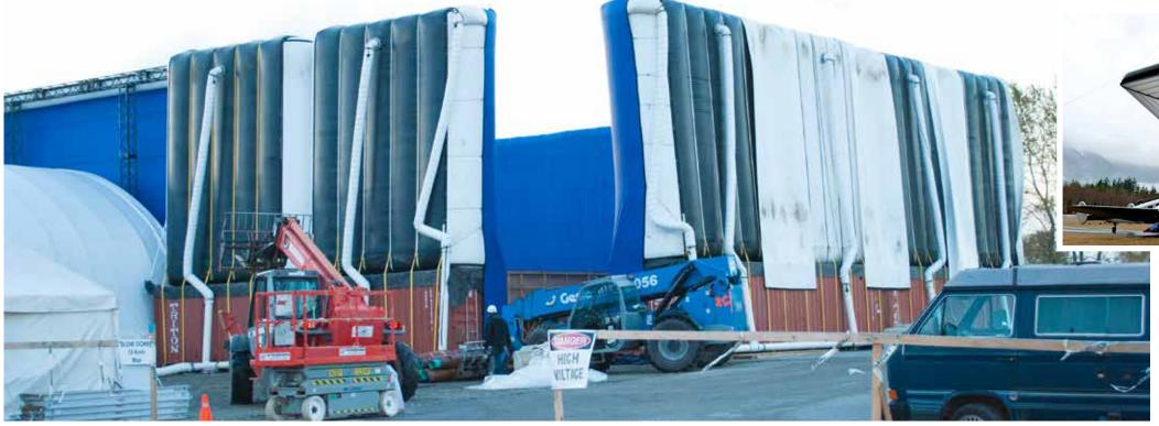
The Airwall comes in sections that are 20ft wide and 24ft tall. Sections can simply be added to reach the required length.
